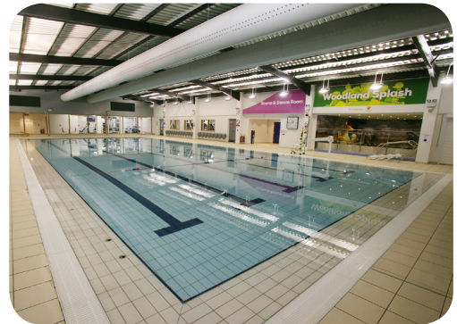
Upgraded pool hall with level deck pool edge
