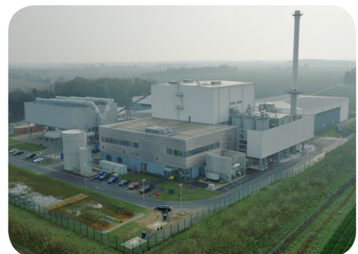
Straw burning power station supplying district heating
