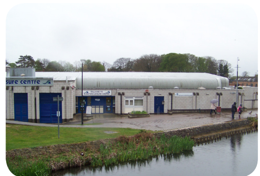
Entrance prior to refurbishment
